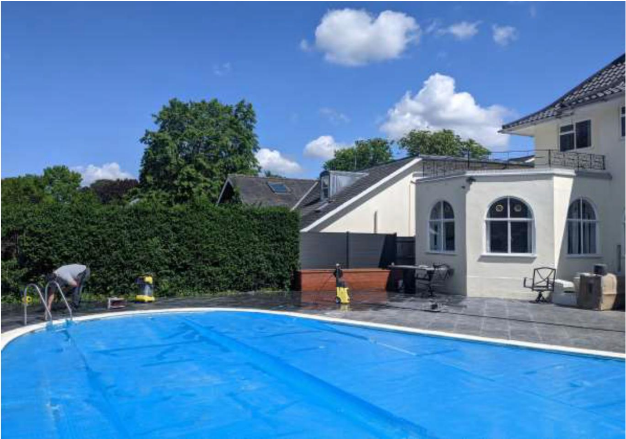
Rear Elevation/View of No. 13 Thornton Grove
